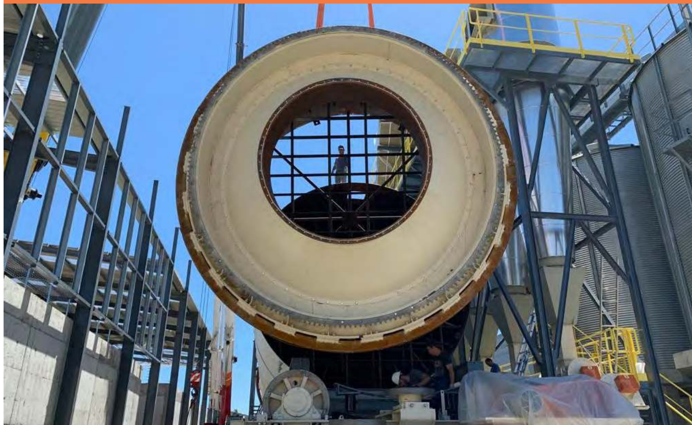
Installation of drying/torrefaction unit. (Source: Futerra Fuels)
